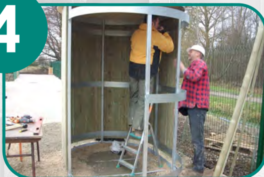
The wooden walls are fixed to the structure
