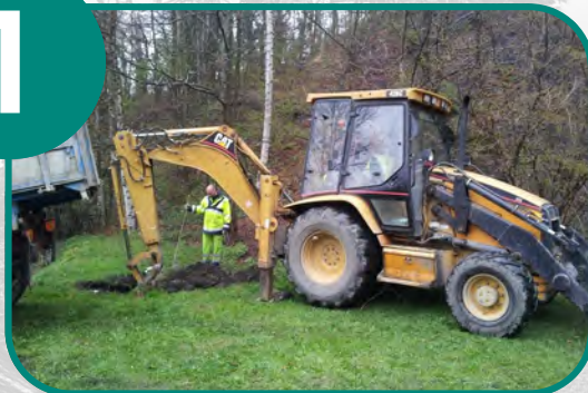
Excavation to install the tank
