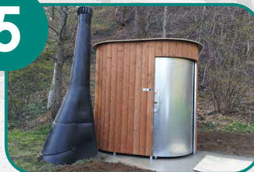
The dry toilet is ready for use
