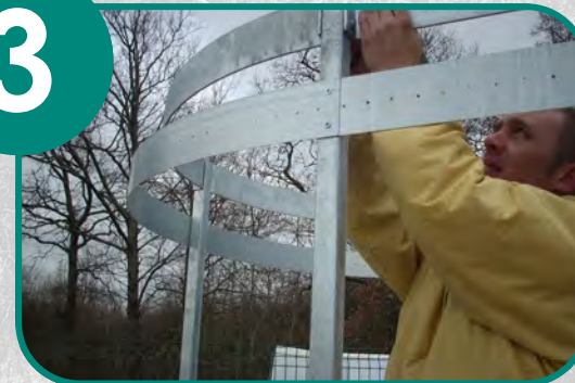
The main structure of the toilet is assembled and positioned
