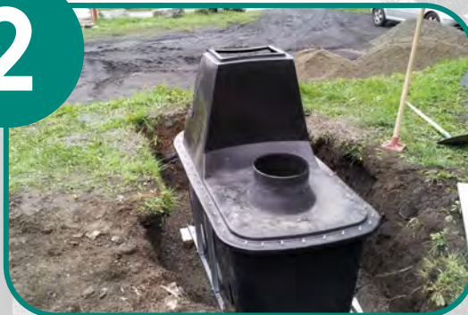
The tank is placing
